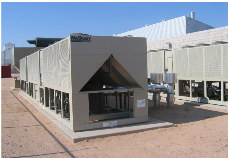
McQuay Genesys Air-cooled screw compressor chillers deliver up to 14 EER at part load and use HFC-134a refrigerant with no ozone depletion or phase-out date.
